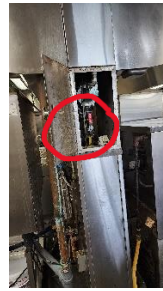
Gas Shut Off picture in main kitchen
